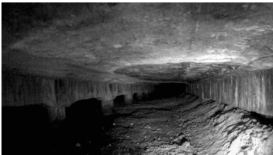
Figure 5b. Under the road surface of the Schoolstraat. To the left, in the middle of the road, the concrete top-pieces on the wooden piles are clearly visible (Photography: Ronald van Gelder, 2013).
