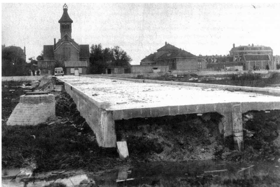
Figure 5a. The Paulus Emtinckweg (one of the roads built on sunken piles) under construction in 'De Nieuwe Buurt'. In the background is the crossing Burgemeester Van Tienenweg (built on sunken piles in 1934), behind which the back of the Sint Petrus Banden church can be seen (1910); on the right of the photograph, parallel to the Emtinckweg, are the Schoolstraat (constructed in 1934) with the Sint Petrus school and on the other side of the road, houses. Visible sticking out above the houses is the roof of the former town hall of Diemen (1882). (Photography: Jan de Boer, 1934) For details on the location of the streets, see Figure 6.
