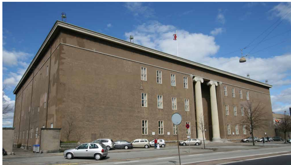
Fig. 5b: The headquarters of the Grand Lodge of the Danish Order of Freemasons, Blegdamsvej, Copenhagen. Photo: Ib Rasmussen 2007.
