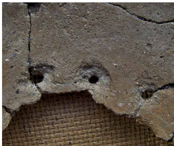
Figure 4.21 Dalfsen: Perforations seen from the inside (AB71).
