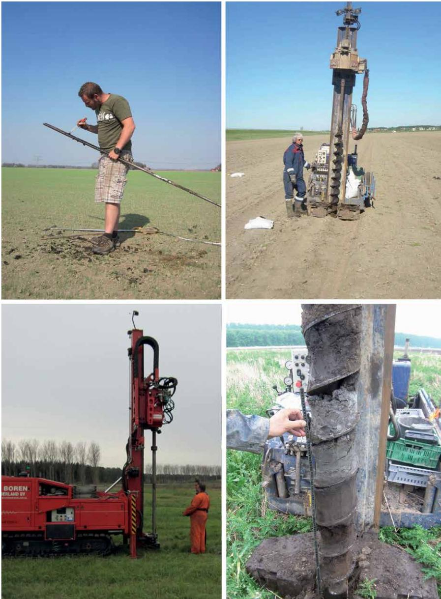
Figure 3.14: Impression of techniques used during borehole surveys in Flevoland. Top left: manual auger; top right: mechanic sonic aqualock drill; bottom left: mechanic Avegaar auger; bottom right: detail of an Avegaar sample (source: De Boer & Lesparre-De Waal 2012; Hamburg *et al.* 2014).
