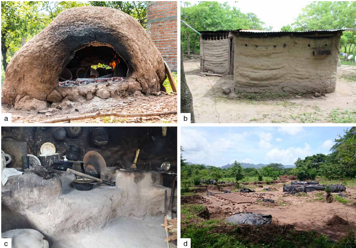
Figure 5: From top left to bottom right: different uses of lanilla soil to build kilns (figure 5a, courtesy of Espora Productions), houses, kitchen ovens (figure 5c, courtesy of Alejandro Arteaga), and an example of a brick manufactory.
