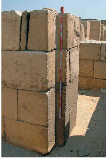
3.6. The tomb of Niankhba: pattern of masonry in the doorway between Rooms E and G.
