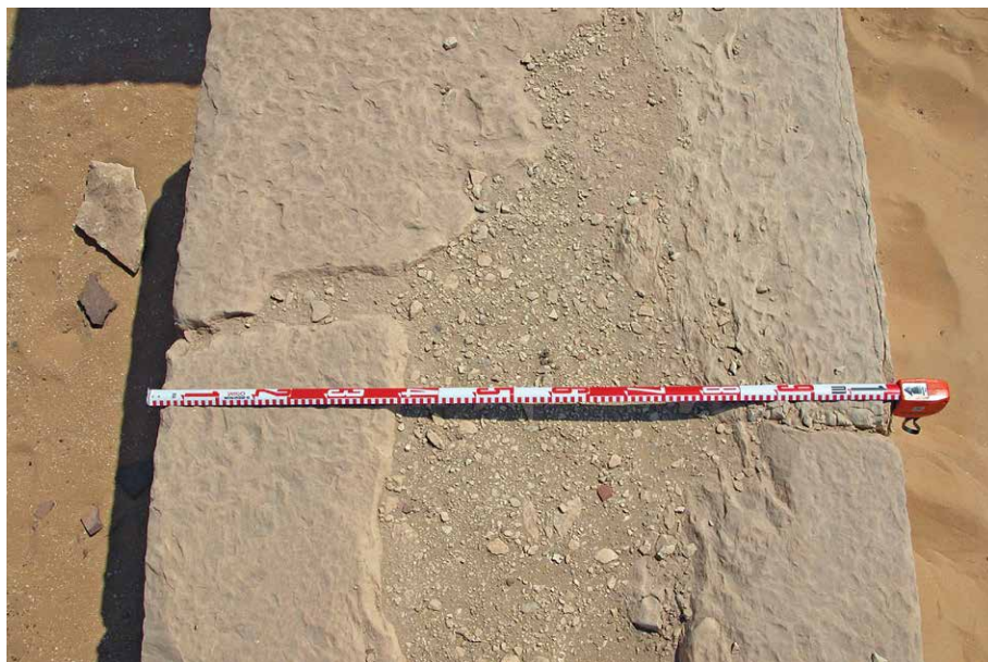
Figure 3.36. Cross-section of masonry within a mastaba in the Unas Cemetery (the tomb of Niankhba).
