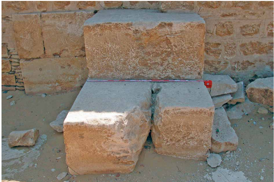
Figure 3.38. Cross-section of masonry within a magazine in the pyramid temple of Unas.
