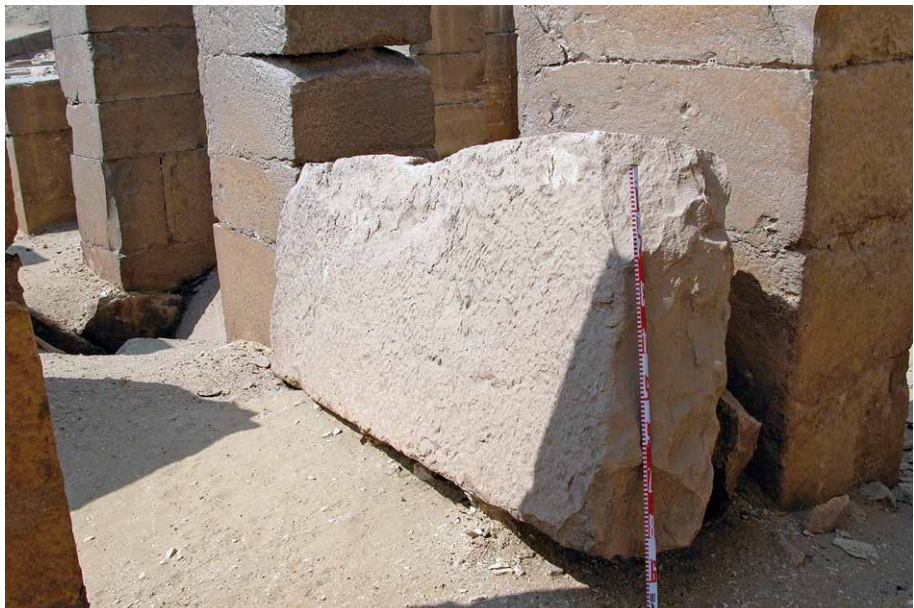
Figure 4.4. The tomb of Niankhba: fallen roofing slab in the columned hall.
