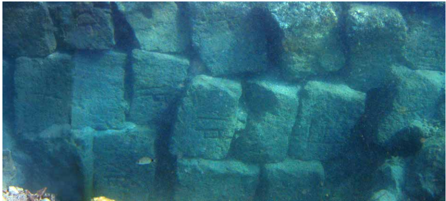
Figure 5. Quarrying and masons' marks on the inner facade of the southern wall. (Photo I. Nouredine).
