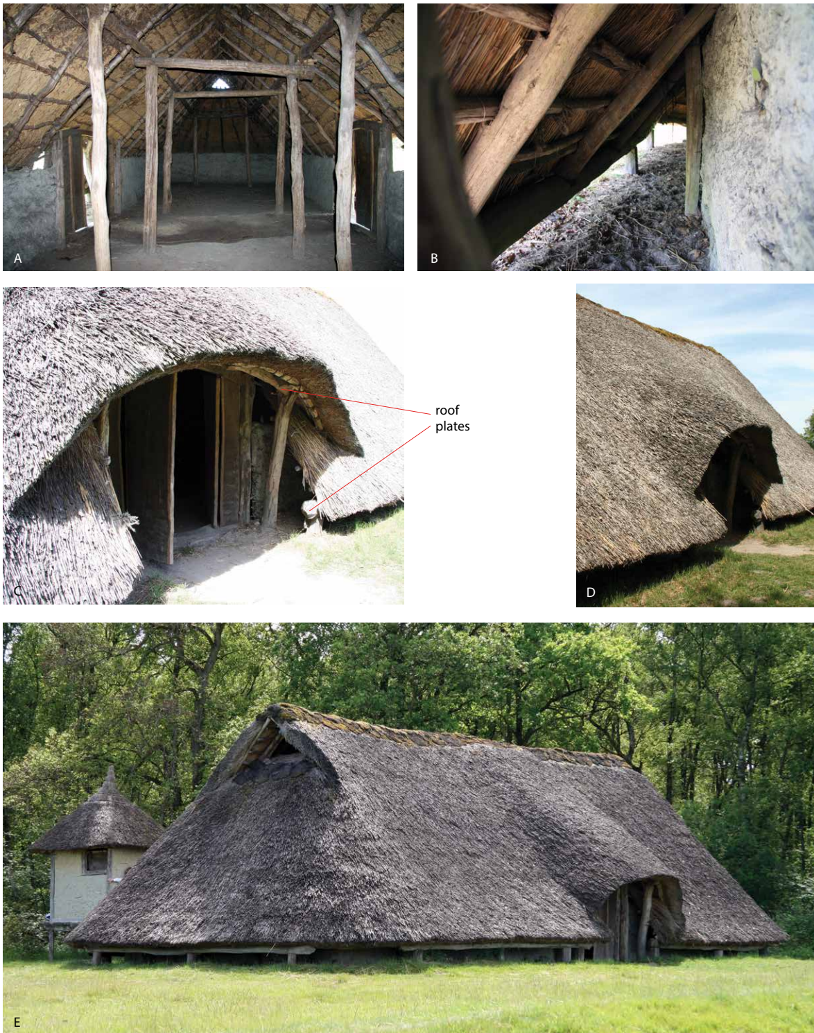
Figure 3.4 The Early Iron Age house reconstruction at Orvelte. All photographs are taken in 2009. A The interior with a portal construction. The position of the mid-beam and the rafters is well visible; B the eaves and the roof-plate resting on the eaves posts; C, D, E raised roof plates above the door. Photo H. Fokkens.
