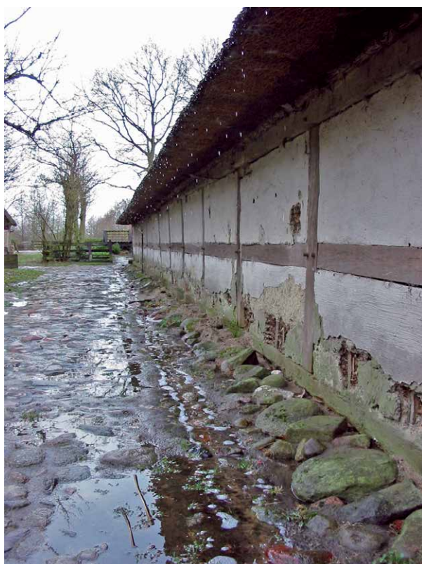
Figure 3.3 Rain water dripping from the eaves and the damage that this does to the lower sides of the walls. Photo taken in Orvelte in 2003 of a preserved historical farm. Photo H. Fokkens.
