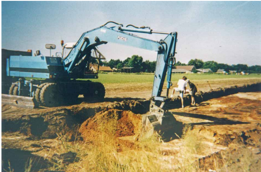
Figure 3. The 'excavation' in 1995 had to be carried out under difficult circumstances (photo G. Smits).
