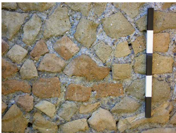
Figure 11.3d: Horrea, via degli Aurighi (III.ii.6). Rubble facing of dividing walls (photo: Janet DeLaine).
