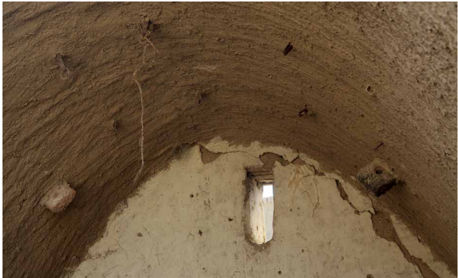
Figure 6: Interior of vaulted room in the village of Bāb with metal loops and fired bricks for hanging up supplies (L. Fliesser © Austrian Archaeological Institute).
