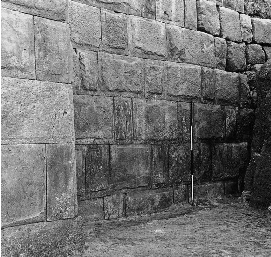
Figure 48.7 Part of the east façade of the stone curtain wall of the Halzi Gate, seen from the east. Note the well-dressed masonry of Tower 3 and the comparable quality of most of the masonry in the adjacent wall-face. The decidedly rougher stonework that lies above and to the right of the 2 m scale is likely to be representative of a late, hurried repair. Note also the white, plastered ground surface that extends outwards from the base of the wall.
