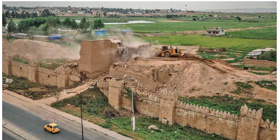
The destruction of the Maški Gate in 2016.
