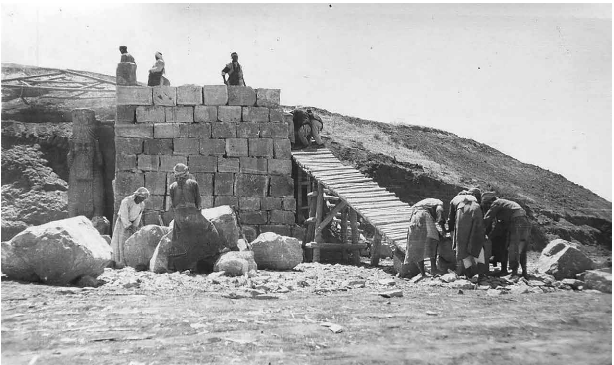
Figure 17.2 Renovation activities at the Nergal Gate in the 1950s.
