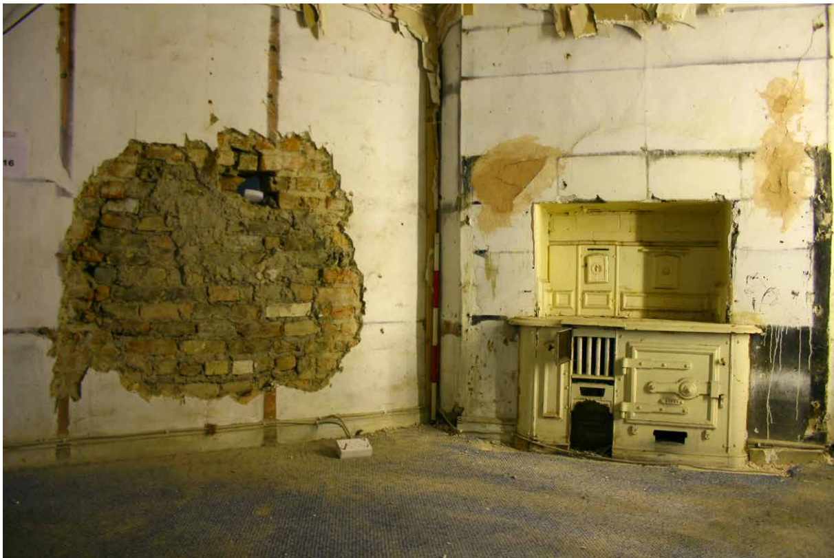
Fig. 5.2. Wall breakthrough through the interior walls of the house at No. 17 Moore Street to No. 16 Moore Street, Dublin, Ireland (© Frank Myles, Archaeology and Built Heritage, 2012).
