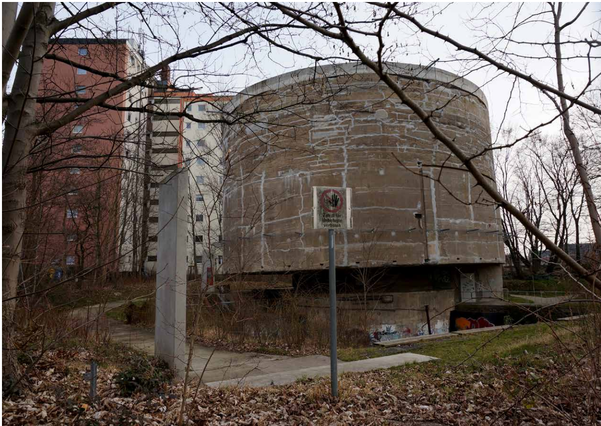
Fig. 12.1. Berlin, heavyweight cylinder ( Schwerbelastungskörper ) to test the stability of the subsoil (© Claudia Theune).
