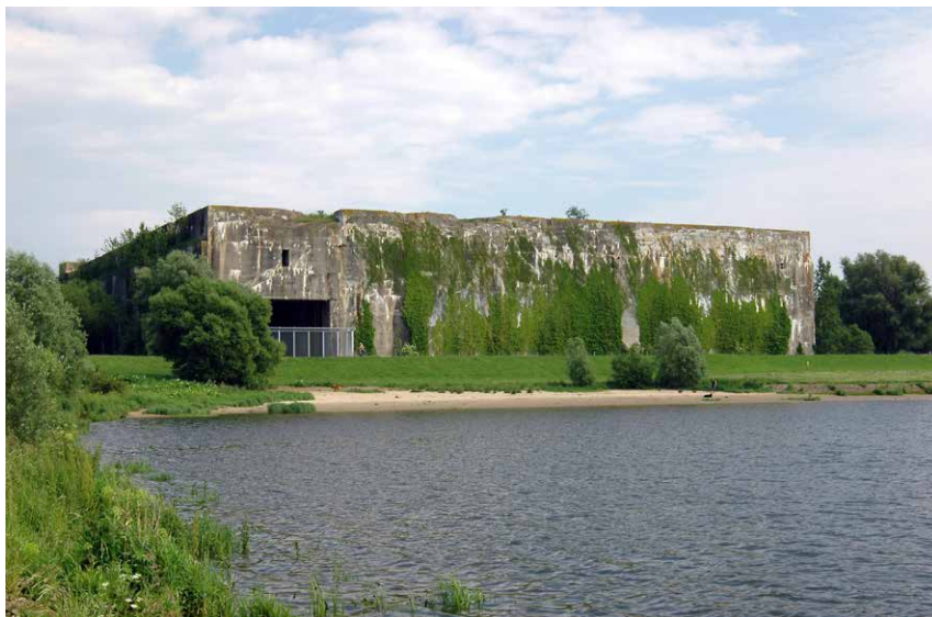
Fig. 4.11. One of the largest bunkers for submarines, the Bunker Valentin, is located in Bremen, Germany (©Landesarchäologie Bremen, photograph H. Steinwand).
