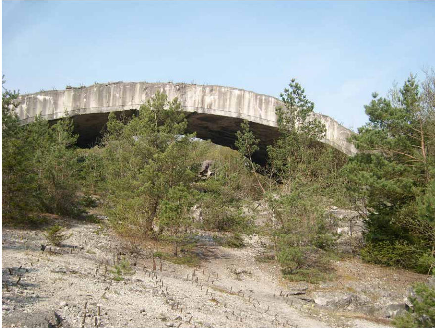
Fig. 4.10. Near Mühldorf am Inn, a semi-subterranean armament bunker for the production of the Messerschmitt Me 262 was built by forced labourers during the Second World War. The bunker measured 33 m wide and 400 m long with eight floors under twelve huge concrete arches. Only seven of the sections were completed. After the war, six of the arches were blown up (© Walter Irlinger).
