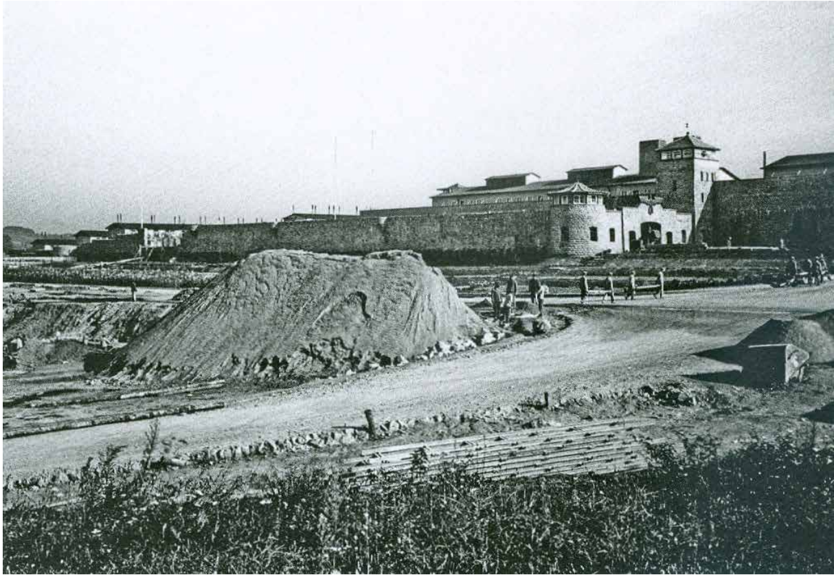
Fig. 6.10. Mauthausen, former concentration camp during the construction works at the so-called Russian Camp / Infirmary Camp; view from south (© MHC Fons Amical de Mauthausen).
