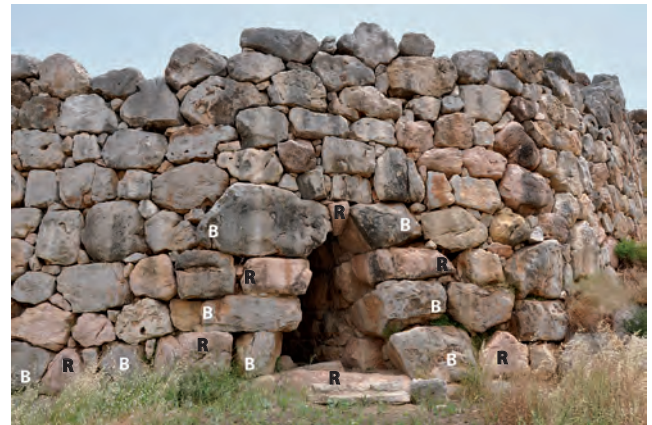
Figure 9 Tiryns Western Staircase indicating intentionally alternating employment of lithofacies E with at least one grey limestone; B=grey, R=red
