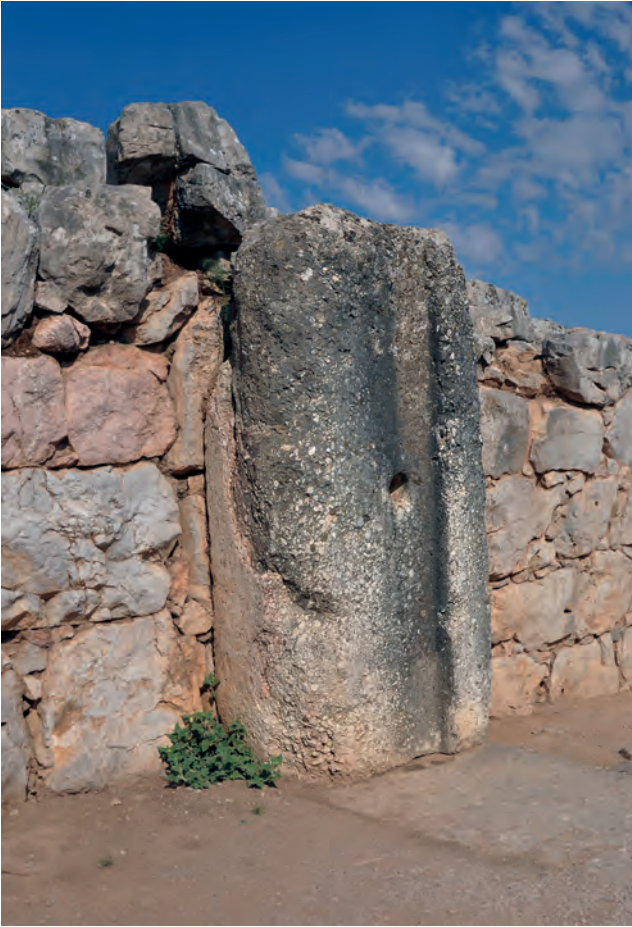
Figure 6 Tiryns east side of the citadel, Great Gate: badly flaking conglomerate upright post
