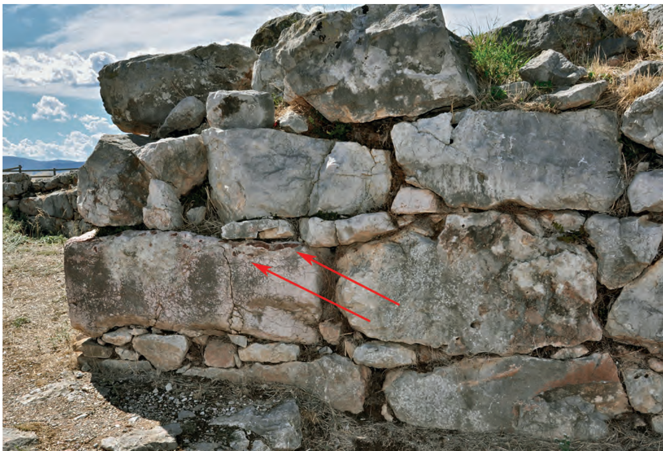
Figure 3 Lithofacies E block showing inclusions of chert and a nodular look caused by veinlet running perpendicular to the stylolites, giving the stone its less robust character
