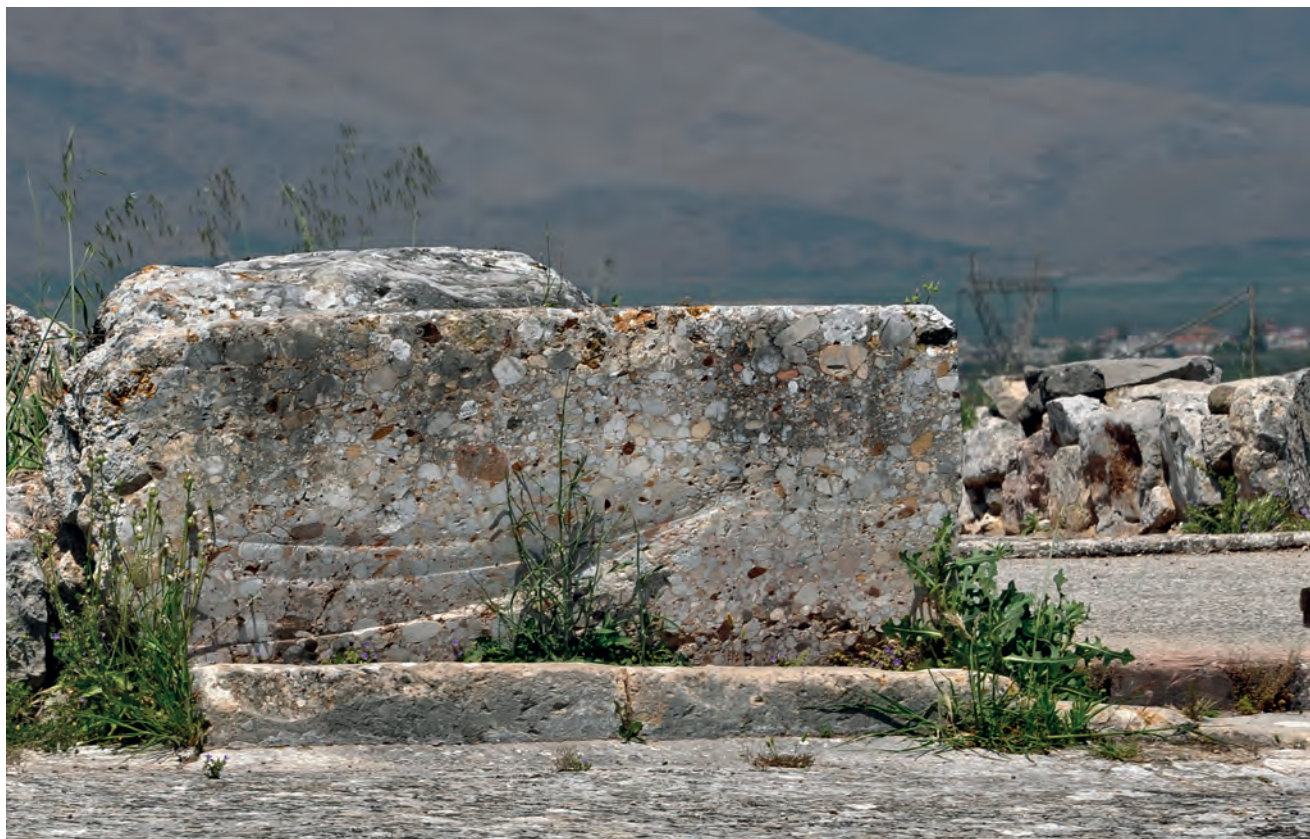
Figure 7 Tiryns upper citadel: conglomerate sawn antae block, left from the low steps leading into the Great Megaron complex
