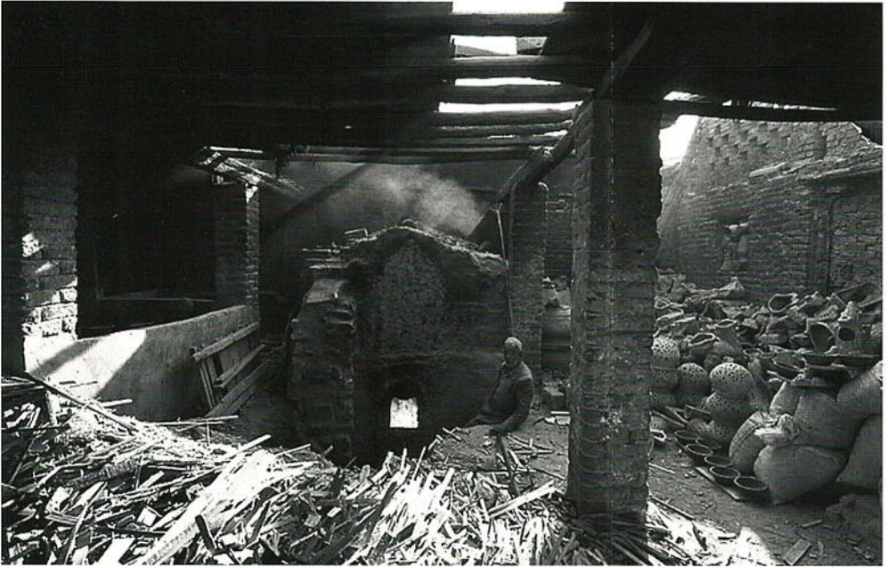
Figure 10. Workshop 2: room 3. A small updraft kiln constructed of stone and bricks.
