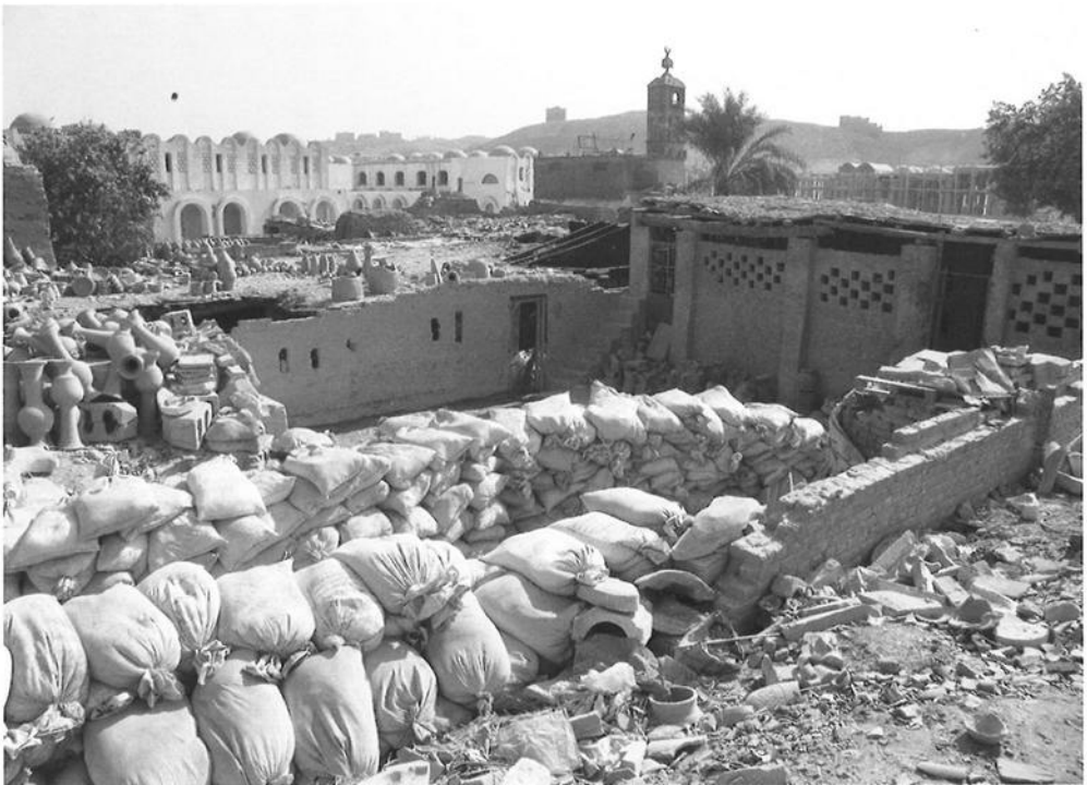
Figure 2. Overview of the roofs of the pottery workshops in Batn el-Baqara, Fustat, looking towards the south-west. The small mosque where the Fustat Pottery Association holds office can be seen in front of the new workshop buildings by the government.
