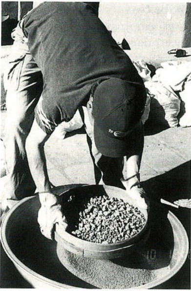
Figure 4. Sieving crushed clay.
