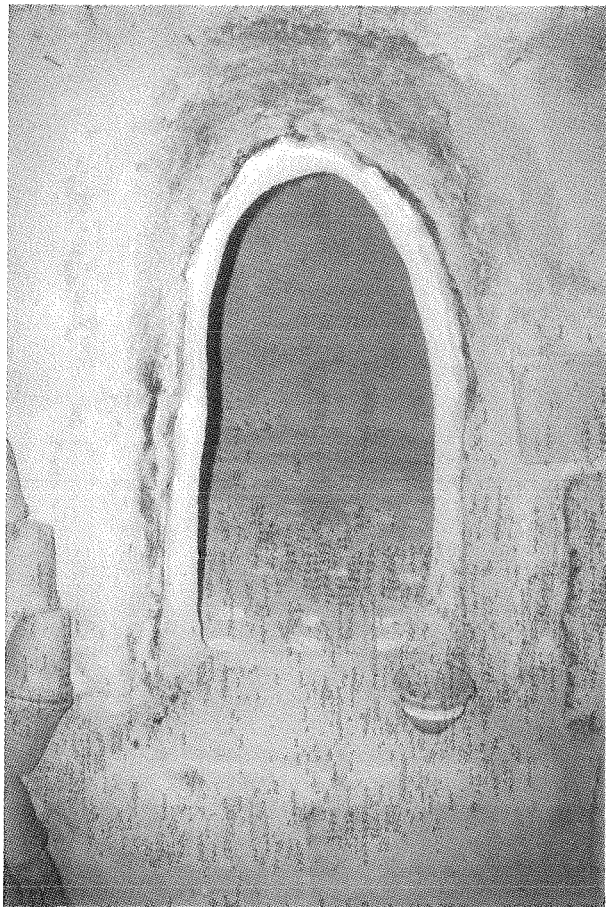
Fig. 3. The pottery chamber of the up-draught kiln.
