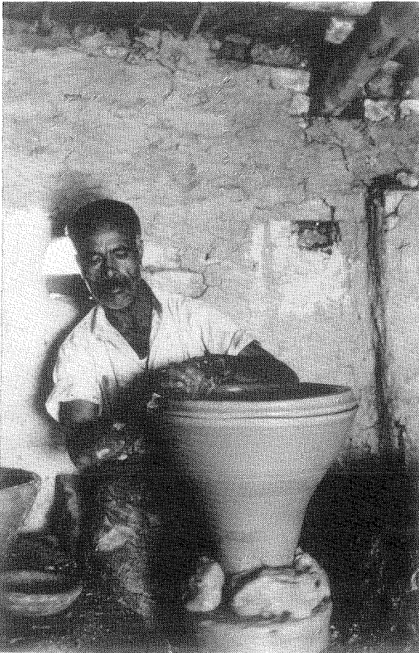
Fig. 6. Throwing the upper part of a water jar.
